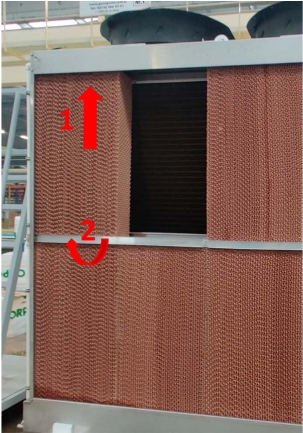
3. In adiabatic cooling system support parts installed. This part generally sends installed from our factory. If It's not, the cooling system has to installed before replace. After, with the help of forklift and crane It passing from product carrying lifting eye is place on support legs and makes top connections of product.
