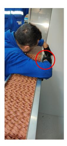
5. lower support sheets places of adiabatic cooling system for supporting
